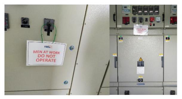
Proper LOTO (Lockout-tagout) system is ensured so that dangerous machines are properly shut off and not started up again prior to the completion of maintenance or servicing work.
